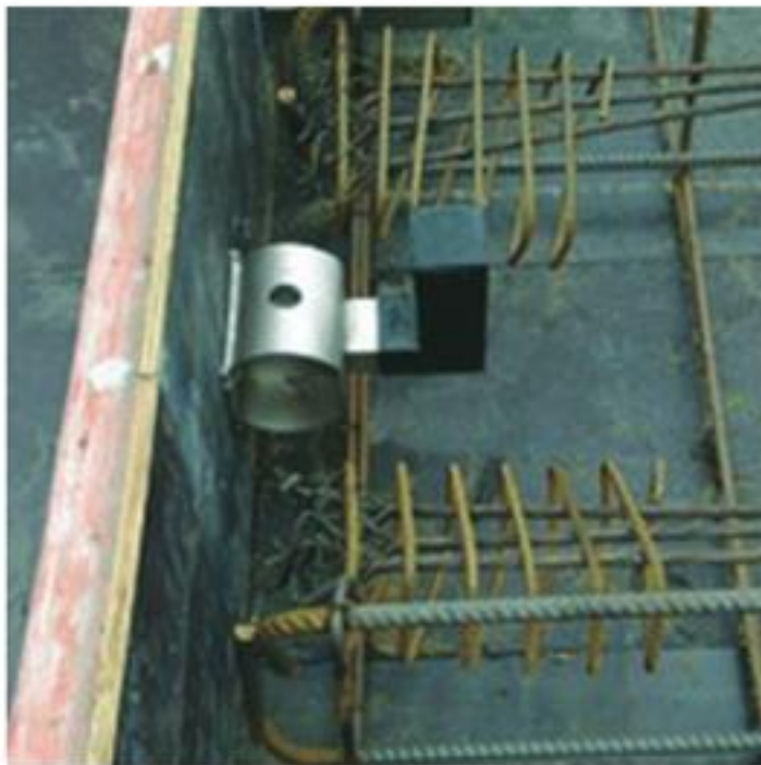
HLDQ-L30 Sleeve nailed to formwork
