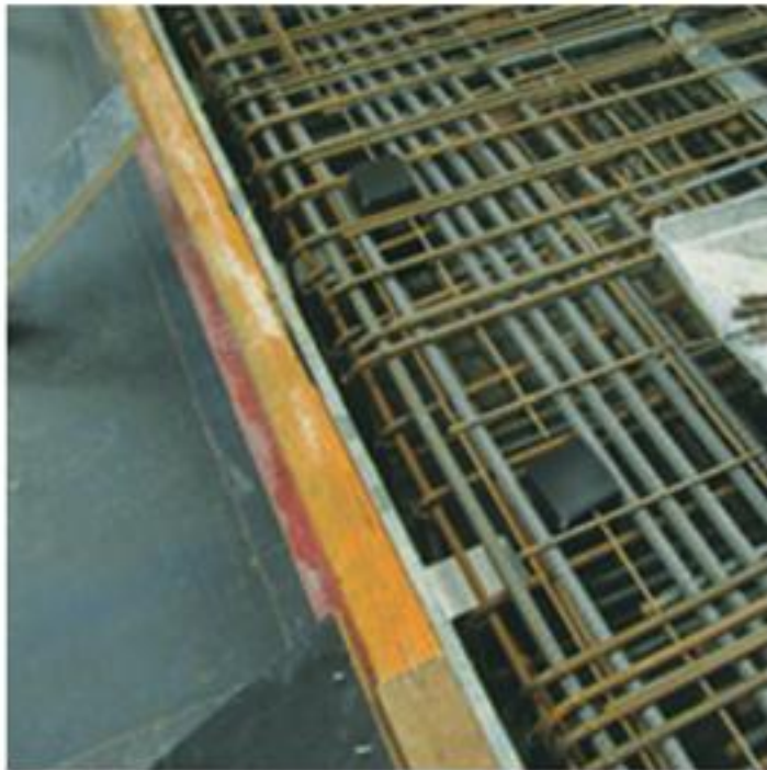
Reinforcement being located around ESDQ-L20 Sleeves
