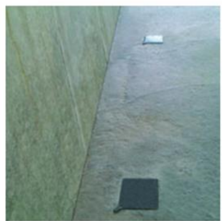
Void formers shown at Slab-to-Wall joint
