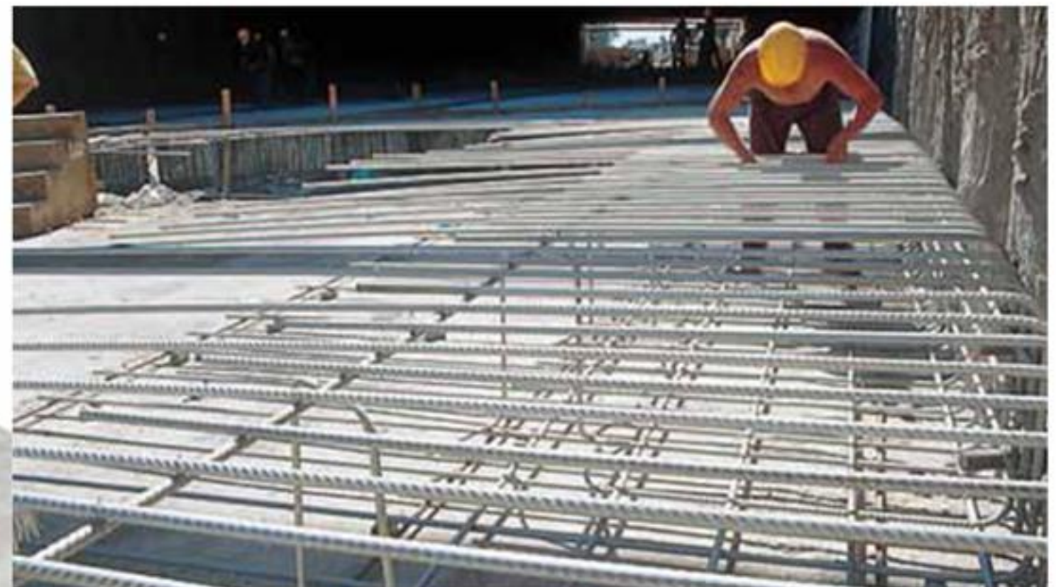
Engineered Reinforcing Bar. Project: Cradlewell Bypass, UK (Contractor: Alfred McAlpine/Carillion)
