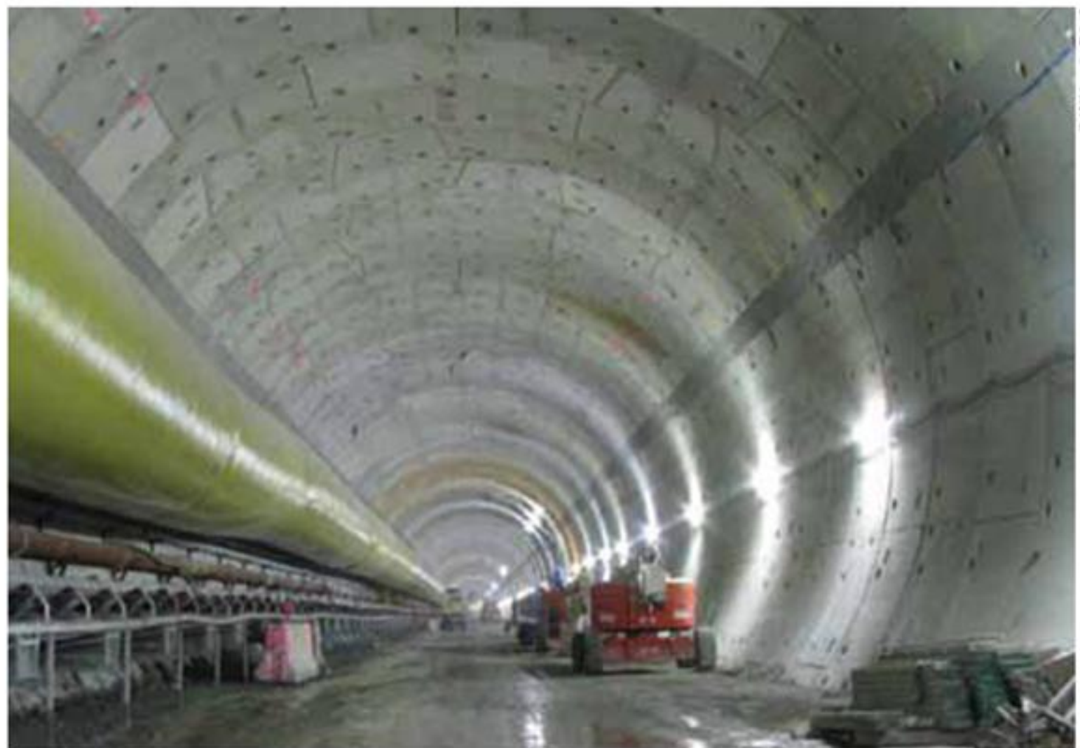
Project: Brisbane North-South Tunnel, Australia (Contractor: LBB JV, Engineer: Bilfinger Berger)
