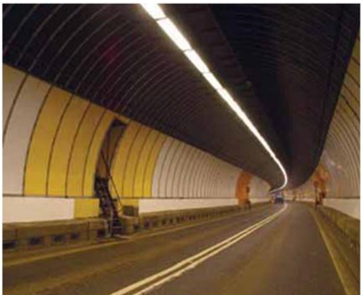
Tunnel Linings. Project: Clyde Tunnel, UK (Contractor: Byzak, Engineer: Faber Maunsell)
