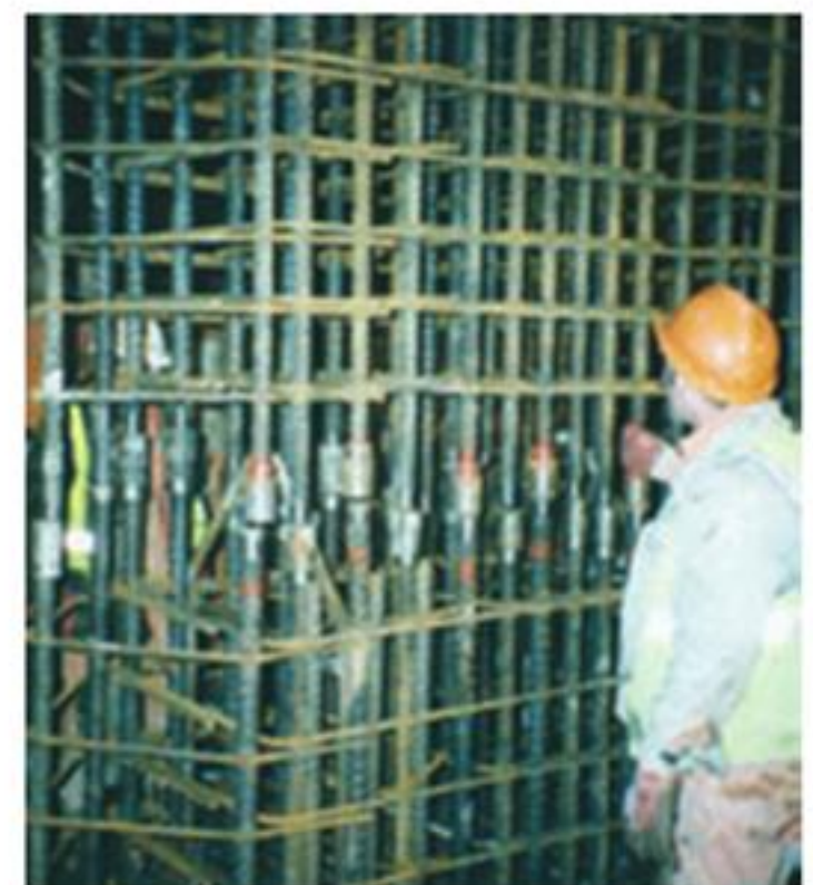
3 Rotate the coupler from the continuation bar to engage against the rear of the thread on the opposing bar and lock tight.
