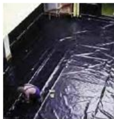
Root Barrier being installed
