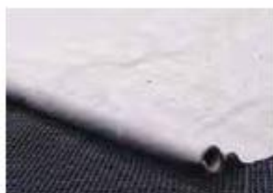
The filter sheet rolled out over the drainage layer
