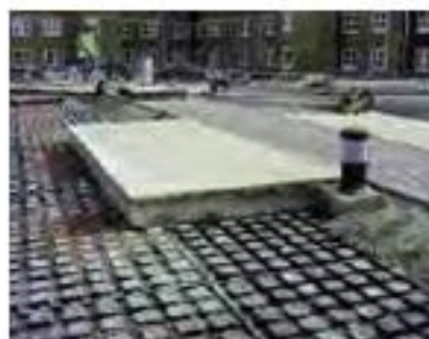
Hard landscaping constructed before substrate layer installed
