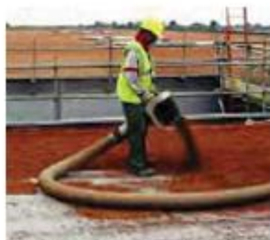
Substrate being pumped in position on a large roof
