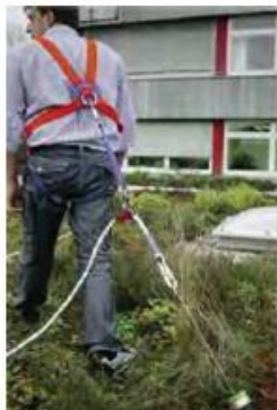
Fig 20: The Fallnet system
