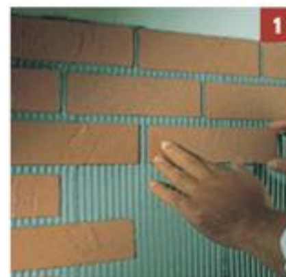
Applying the brick slips
