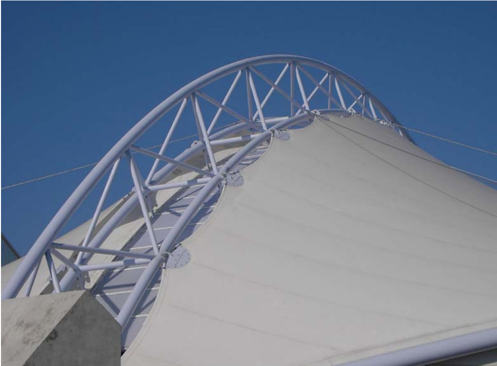
Exterior view of Chatham structure. Roof achieved U value of 0.2 - 0.25 W/m 2
