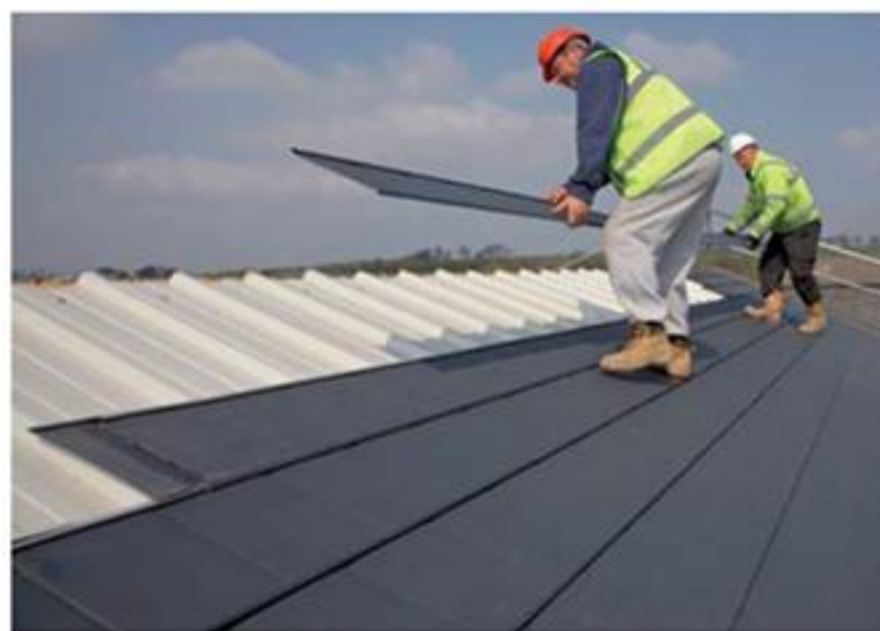
Below and right: Carnwood Park, Leeds. Meta-SlatePlus roofing system with barrel rooflights to a new building during and after installation with view from inside showing underside of AS35 panel.
