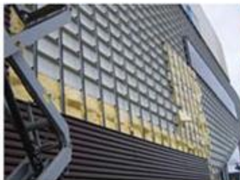
APL StrongBak™ – the most cost-efficient SFS system – the quickest complete closure and airseal of a building
