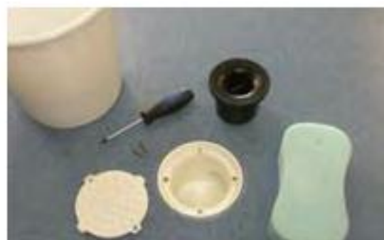
Wash internal surfaces with diluted disinfectant and soft sponge. Reverse process to re-assemble.
