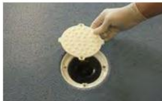
Lift aside Cap taking care not to lose screws. Do not remove Clamp.
