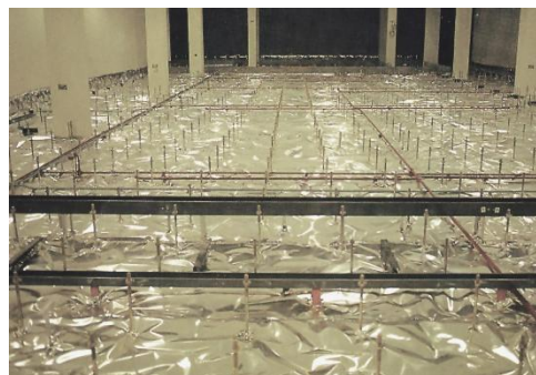
Eco-Brite® installed below under floor heating pipes
