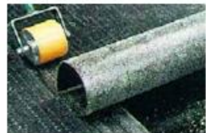
Cold applied Derbiseal S adhesive, pressure rolled using a lap roller.
