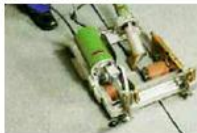
Hot air welded and pressure rolled using a lap roller.
