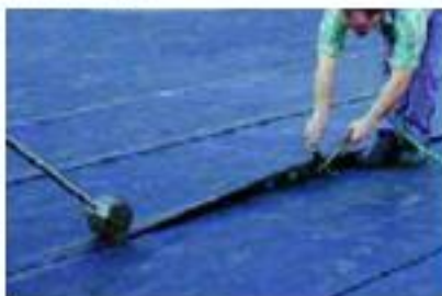
Torch sealed and pressure rolled using a lap roller.
