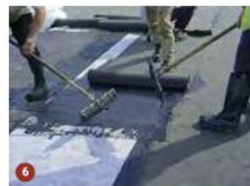
6 Laying Hydrogard Protection Sheet
