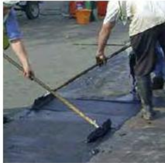
1. Applying the first coat of Hydrotech Monolithic Membrane 6125 with a squeegee
