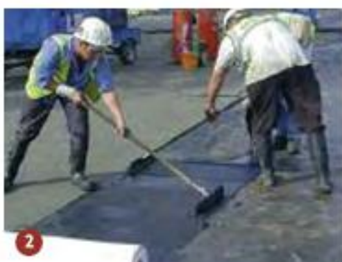
2 Spreading Hydrotech Monolithic Membrane 6125 (First coat)
