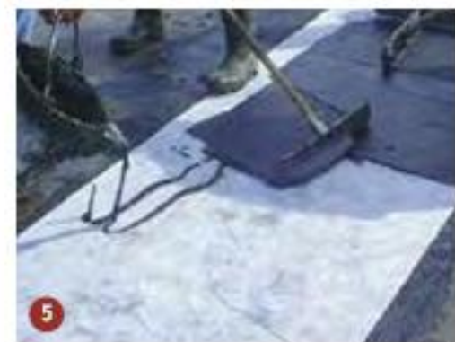
5 Spreading Hydrotech Monolithic Membrane 6125 (Second coat)
