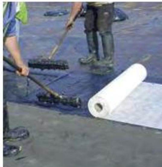
2. Laying Flex Flash F reinforcement
