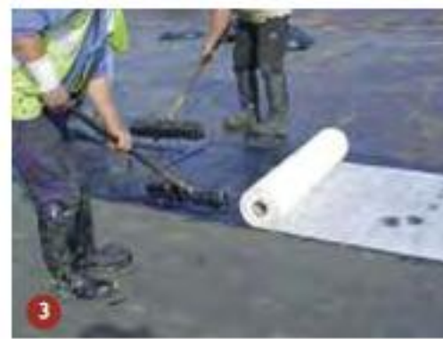
3 Laying Flex Flash F
