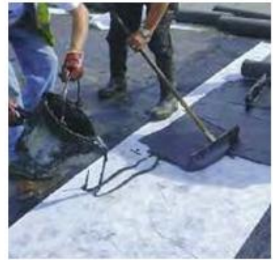
3. Applying the second coat of Hydrotech Monolithic Membrane 6125
