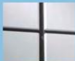
Post-formed panel detail with contrasting flashgap
